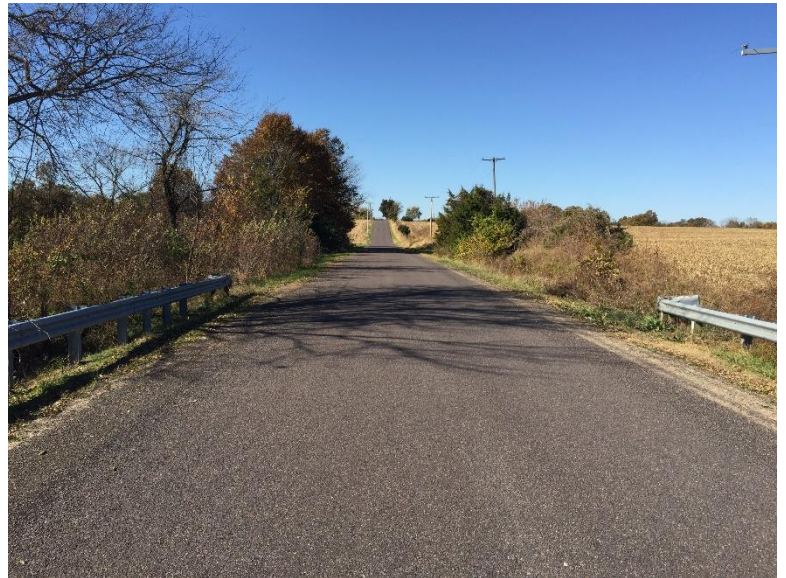
Looking west along Stoenner Road from the structure The roadway is chip sealed with minimal grass shoulders. Roadside ditches get steeper as they approach the structure. Guardrail has been installed.
