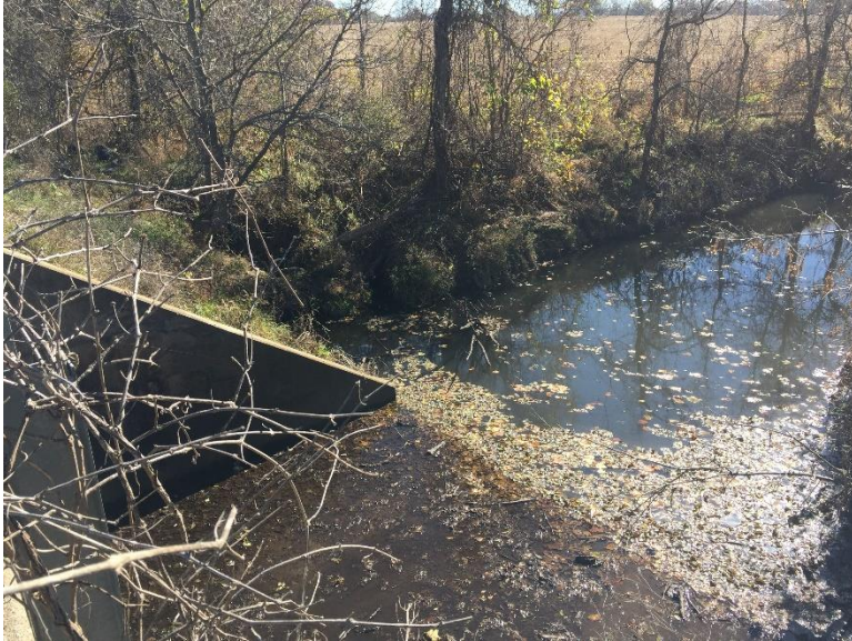
Upstream end of the structure. No center wingwall was constructed. Note the erosion of the roadside ditch at the end of the southeast wingwall. Rock blanket should be considered for each of the locations where the roadside ditches enter the streamway to prevent erosion.
