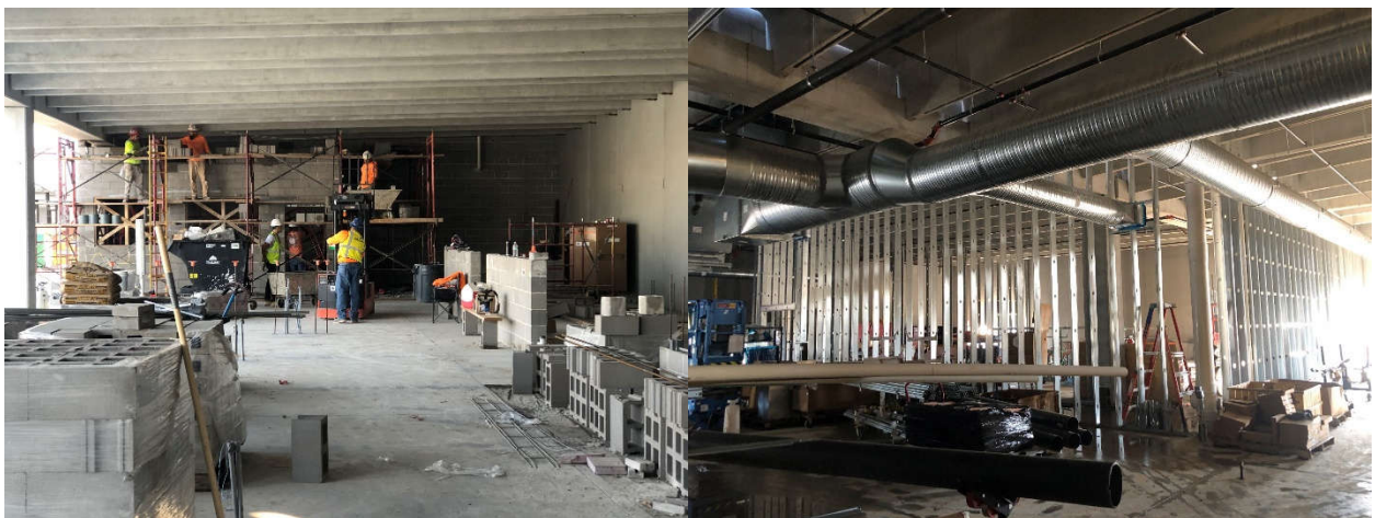
Interior CMU partitions and metal stud partition walls being constructed with duct work overhead.
