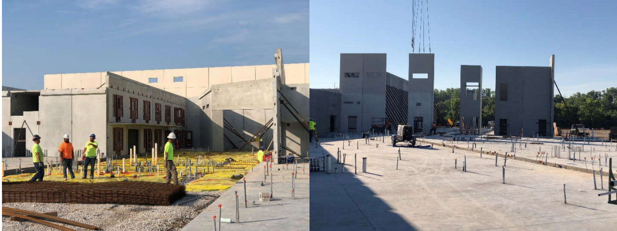
Slab on grade preparation, and precast panel placement.
