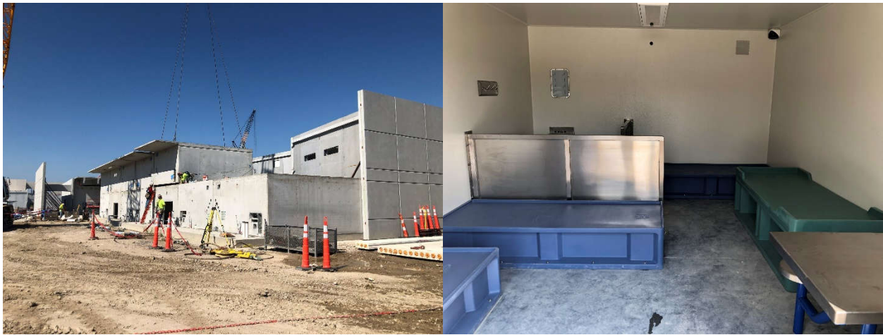
Precast cell modules being placed and an interior mockup.
