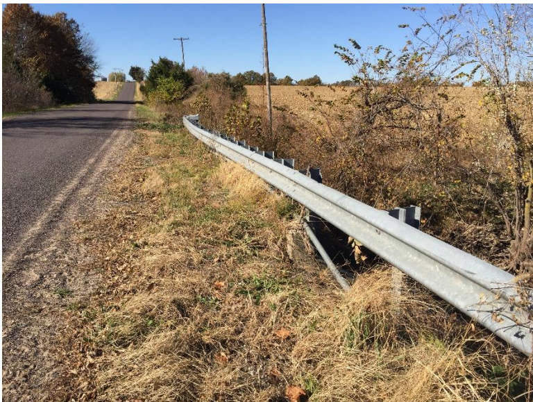
Looking west along the north side of Stoenner Road at the structure. Note the underground utility that crosses over the double cell RCB (assumed fiber optic). During the field visit we noted overhead power and telephone on the poles. We did not see any markers for gas or water at this time. Need to review the County records for private easements.
