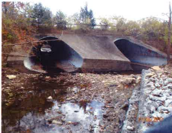
Upstream Elevation Looking Southeast (17'-2" x 11'-4" x 211' Culverts)
