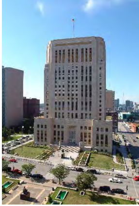
Jackson County Courthouse located in downtown Kansas City, MO.
