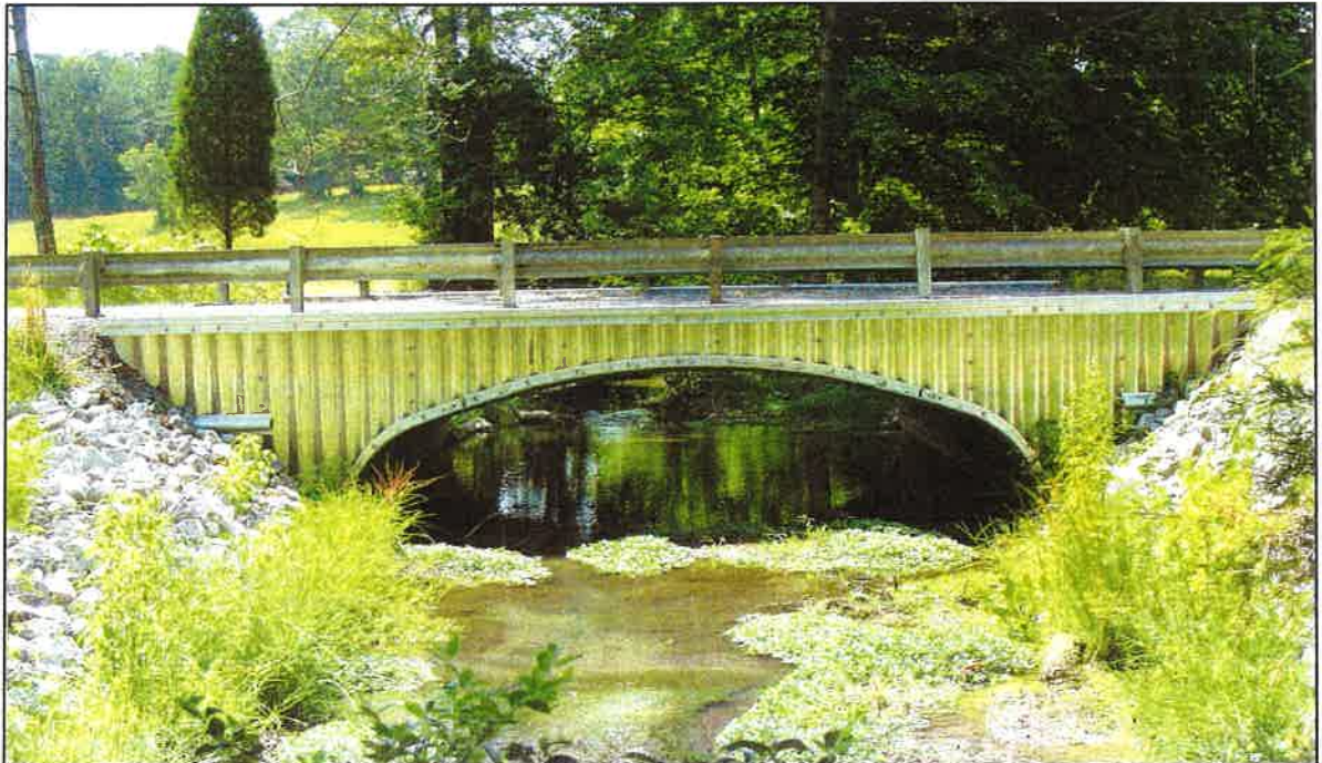
Aluminum Box Culvert - stream crossing
