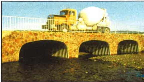
Aluminum Box Culvert - county road bridge
