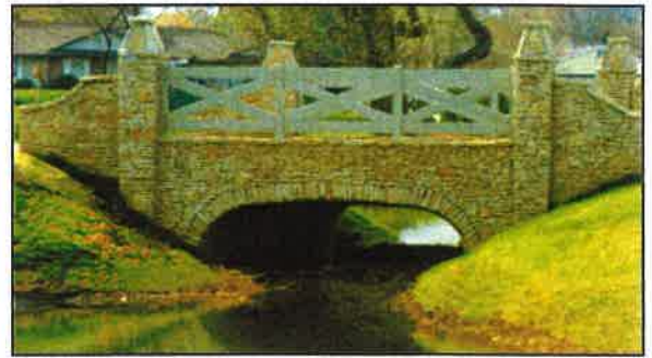
Aluminum Box Culvert - aesthetic finish
