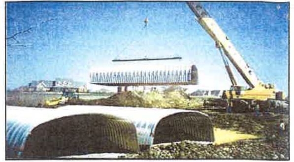
Aluminum Box Culvert - multi-cell installation
