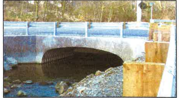
Aluminum Box Culvert - stream crossing
