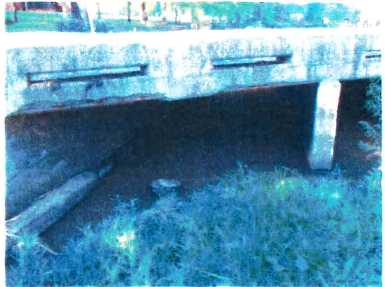
July 2017 site photo of the upstream side of the structure. Note the exposed steel at the bottom of the top slab.
