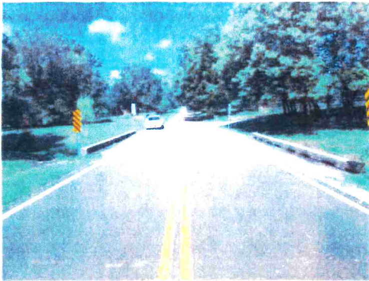
July 2017 site photo looking west across top of the structure.
