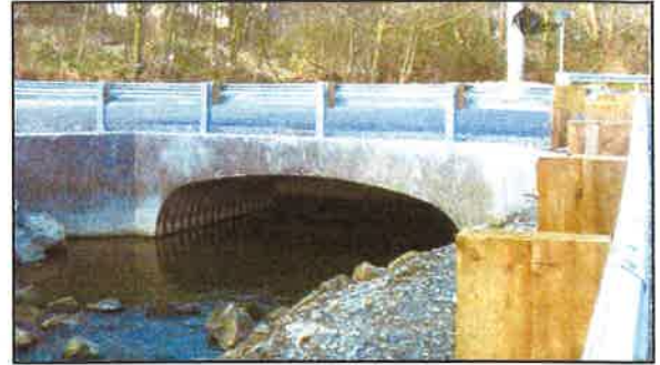
Aluminum Box Culvert - stream crossing
