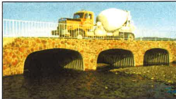
Aluminum Box Culvert - county road bridge
