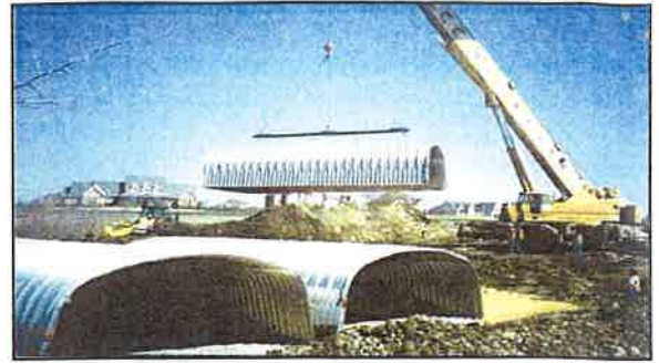
Aluminum Box Culvert - multi-cell installation
