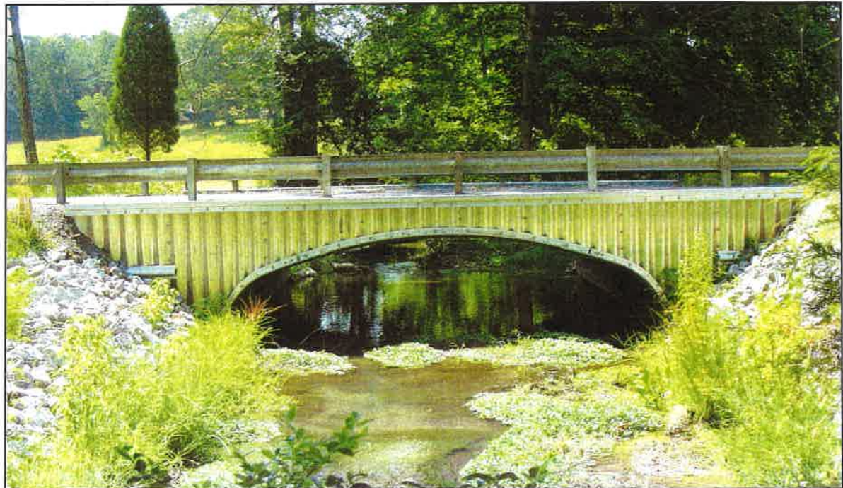
Aluminum Box Culvert - stream crossing
