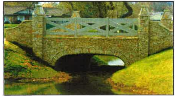
Aluminum Box Culvert - aesthetic finish
