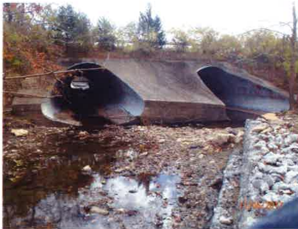
Upstream Elevation Looking Southeast (17'-2" x 11'-4" x 211' Culverts)
