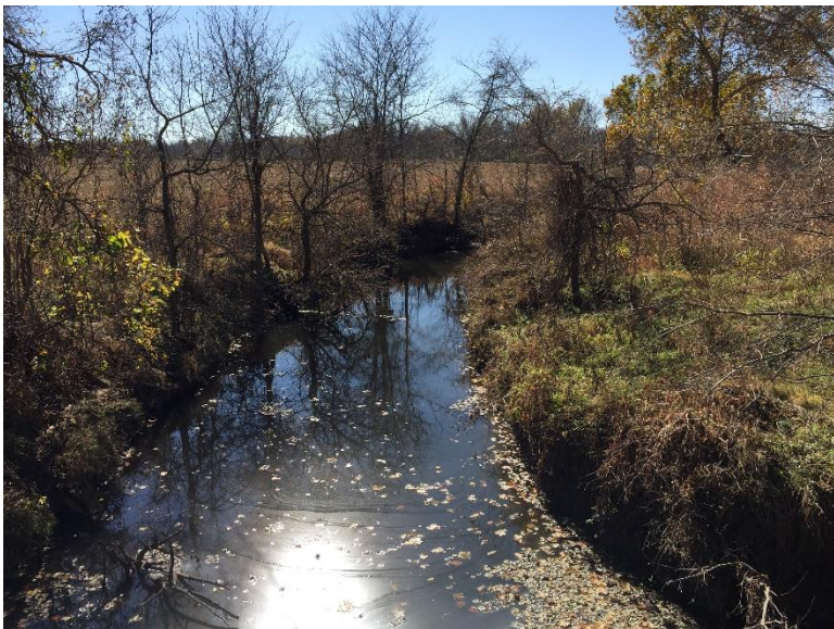
Looking upstream from the double cell RCB. The stream banks are very well defined and extend outside the wingwalls of the structure.
