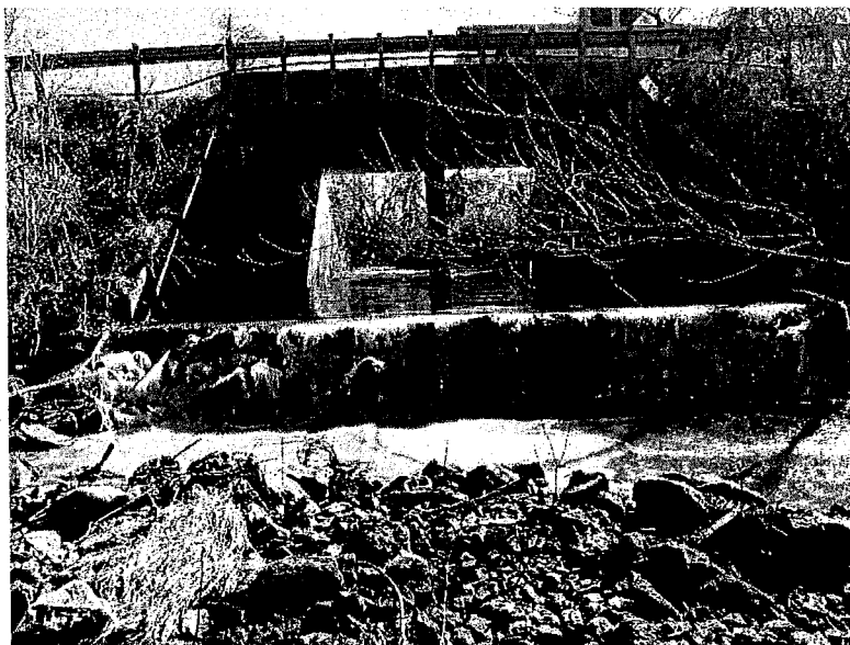
Looking at the downstream end of the structure. There is a significant drop from the end of the apron to the actual stream bottom.
