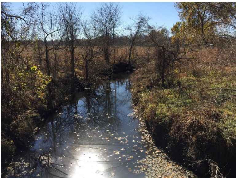
Looking upstream from the double cell RCB. The stream banks are very well defined and extend outside the wingwalls of the structure.
