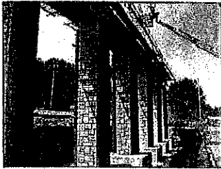
Bridge Columns at Little Blue Parkway
