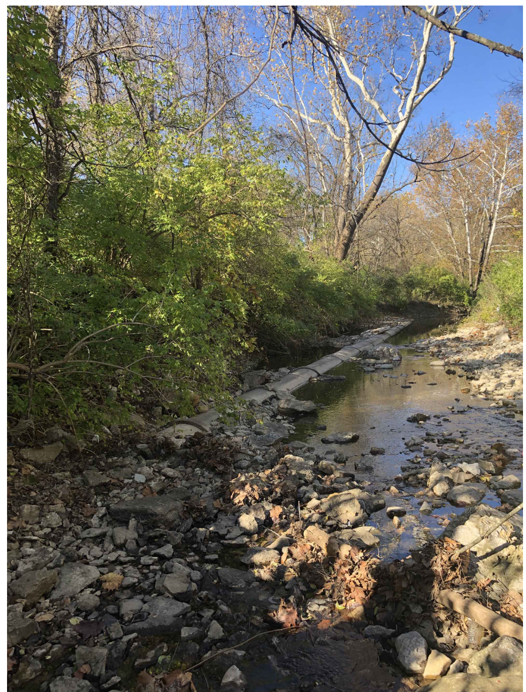
SITE 36 - MH S084-191 LOOKING NORTH
