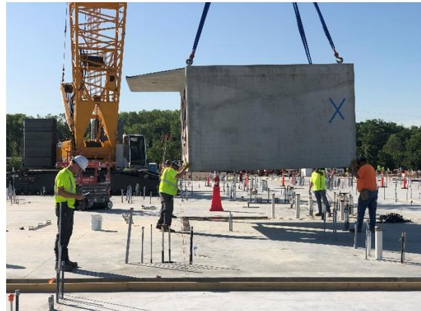
Placement of these units took place over two days however it will take an additional 3 weeks to fully complete their installation. Upon arrival units still require the installation of electrical and plumbing systems as well as paint and interior accessories.
