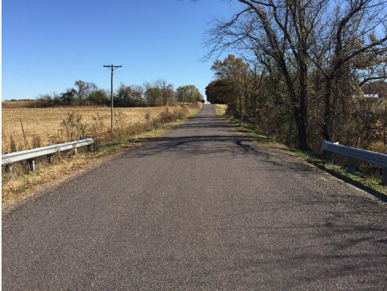
Looking east along Stoenner Road from the structure The roadway is chip sealed with minimal grass shoulders. Roadside ditches get steeper as they approach the structure. Guardrail has been installed.
